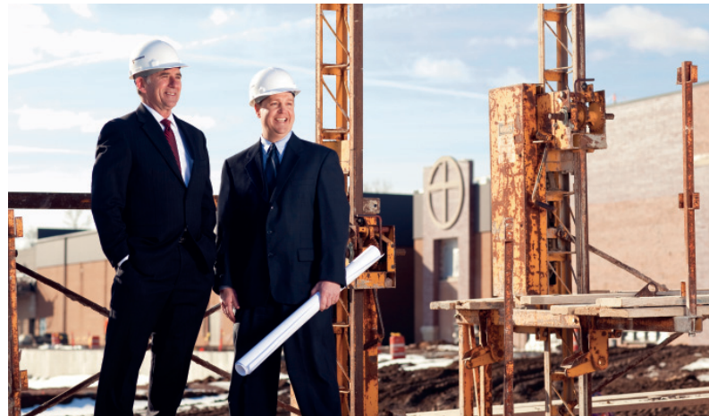
Head of School for Westminster Christian Academy Jim Marsh and Cass Church Banking Advisor Brett Dempsey survey construction progress on-site. A total of $50 million in construction, renovations and improvements is under way in anticipation of the school moving to the new campus in 2011.
